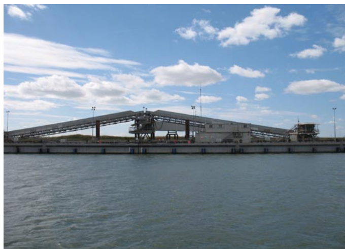
For unloading Crossrail spoil onto Wallasea Island
